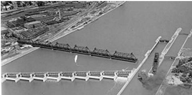
Lock and Dam (1934)
